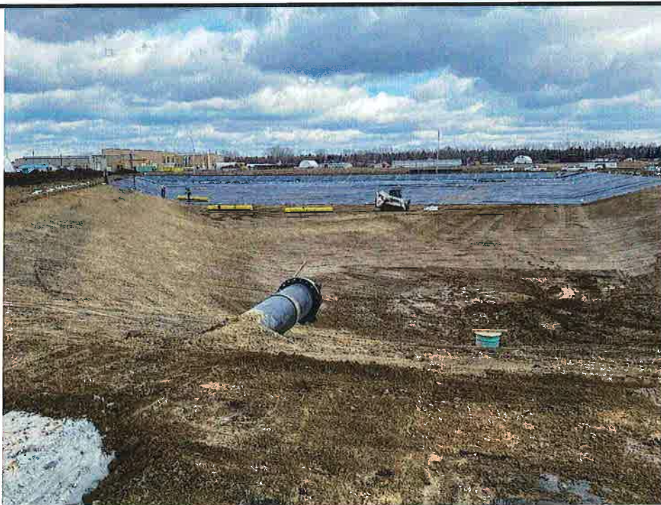
Photo #4 Laying down filter cloth and installing the pond liner
