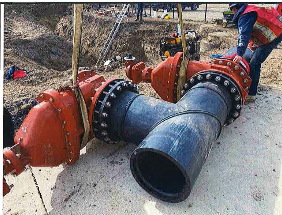
Photo # 3 Valve assembly built ready to be inserted in the line so flows can be diverted out to the storage pond.
