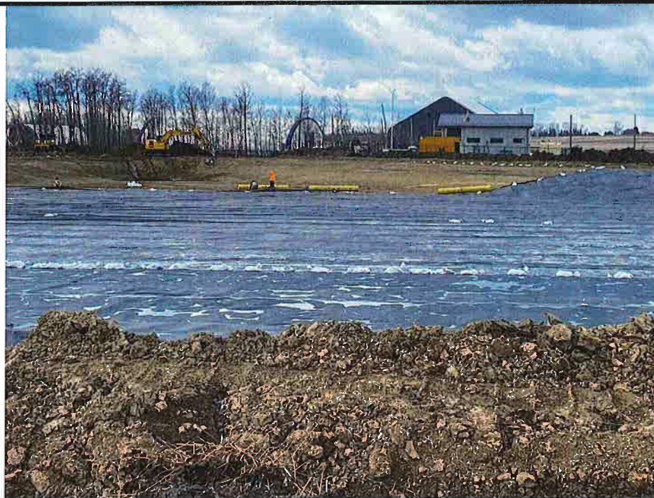
Photo # 3 Pond liner being installed
