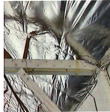
Photo 3: Knee Brace Connection
