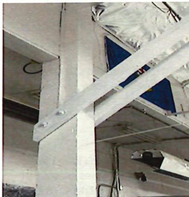
Photo 4: Knee Brace Connection
